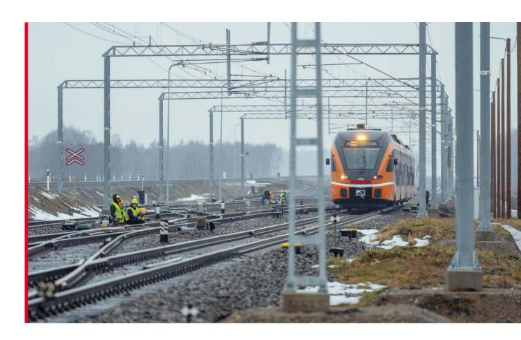
**Straightening Curves and Major Overhaul of the Tartu-Valga Railway Line.** The work involves straightening the Palupere–Puka sections (10.2 km) and a major overhaul of the Puka–Keeni section (11.4 km), the removal of the Puka station, and the construction of 7 culverts. The majority of the work will take place between 2026 and 2027.
